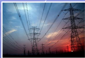
Utility network inspection
